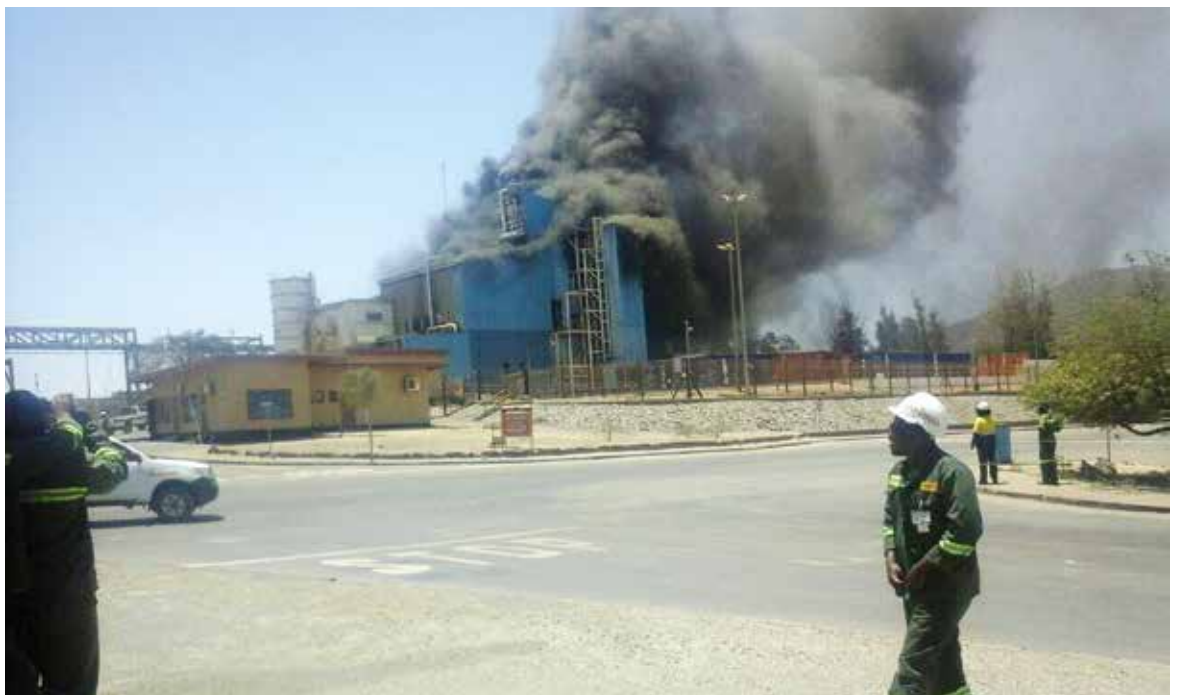
Figure 1: Fire breaks out at FPR in February 2015
